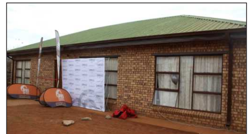
From shack to big house ..... the newly built house for the Nkgadima family.
